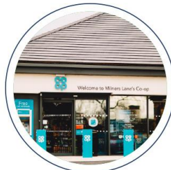
Oct 2016 Telford – Milners Lane New build
