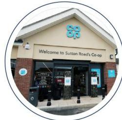
Aug 2016 Shrewsbury – Sutton Road New build
