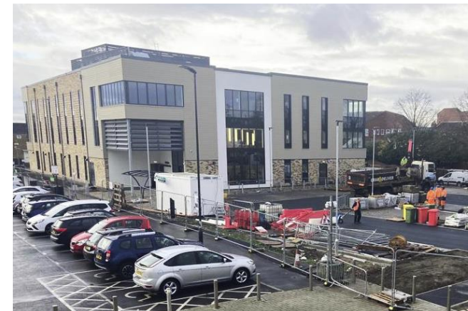
New medical centre, Wallsend
